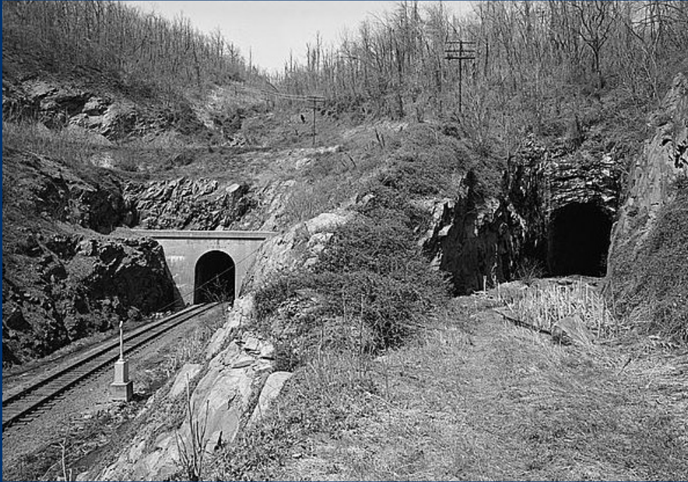
Figure 1. Blue Ridge Tunnel, Afton, Virginia
